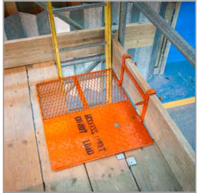
Ladder Safety Hatch - Closed Position
