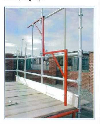
3.3 Attach front of Gate using 120 x 12mm Nut and Bolt.
