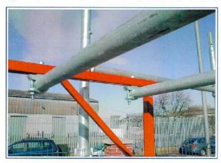
3.5 Finally adjust Gate Position to suit front of Loading Bay.
