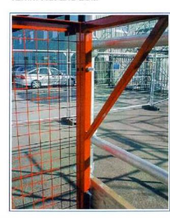
3.4 Fit Ledger Tubes to Back Rail and secure with Scaffold fitting.
